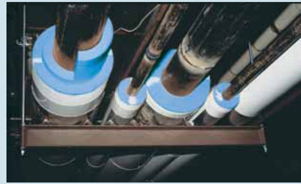
Application of Trymer® pipe covering on a piping network.
