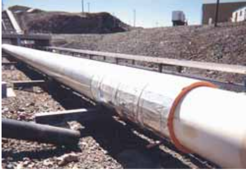
'Wrap-around bevelled lagging system' manufactured by Polybrand from Trymer® foam for a large diameter oil transmitting pipeline.
