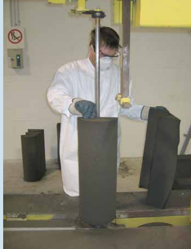
Cutting Foamglas ® pipe covering.
