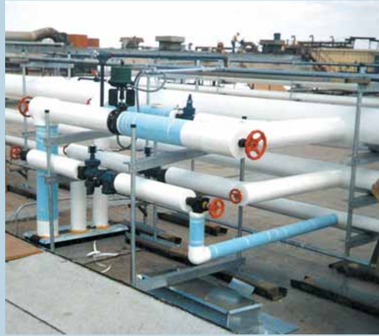
Application of Styrofoam® pipe covering.
